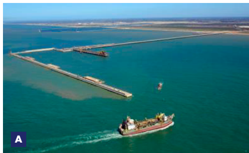
A Aerial view of Terminal T1 B The Project Location C TSHD Prins der Nederlanden
