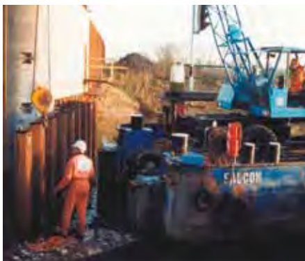
Pulling up sheet piling.
