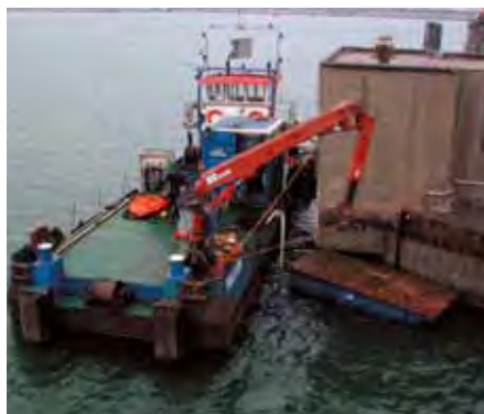
Pulling up sheet piling.
