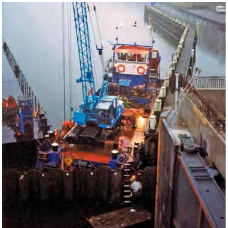
Overhead view of 'Falcon' during activities at the Andel sluice.
