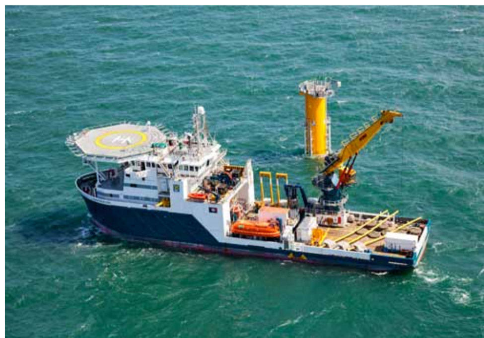
DSV 'Constructor' at work at the Sheringham Shoal wind park, United Kingdom.
