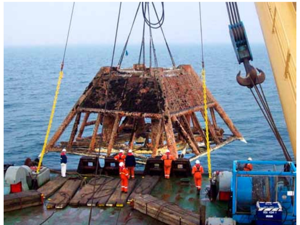
The gas well protection structure lifted to the surface.
