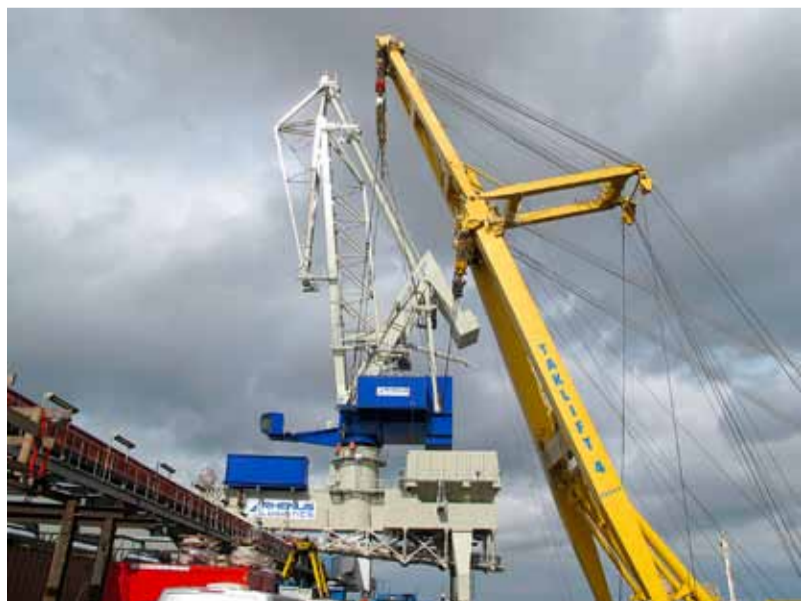
Taklift 4' positioned two crane topsides onto lower crane structures.
