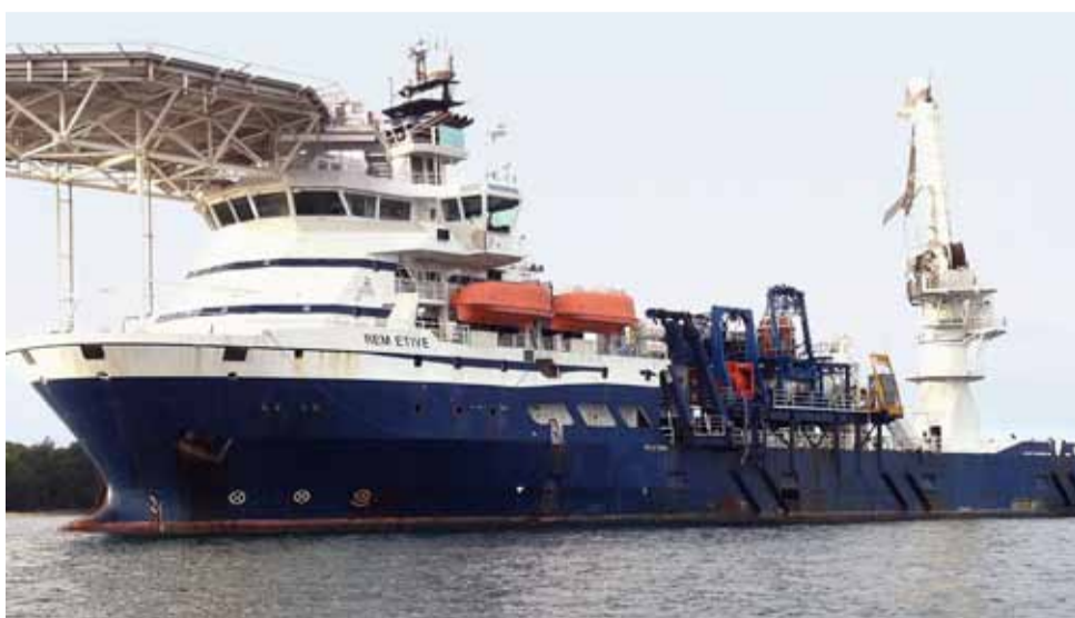
SMIT Subsea's SAT-4 modular saturation diving system on board of the 'Rem Etive'.
