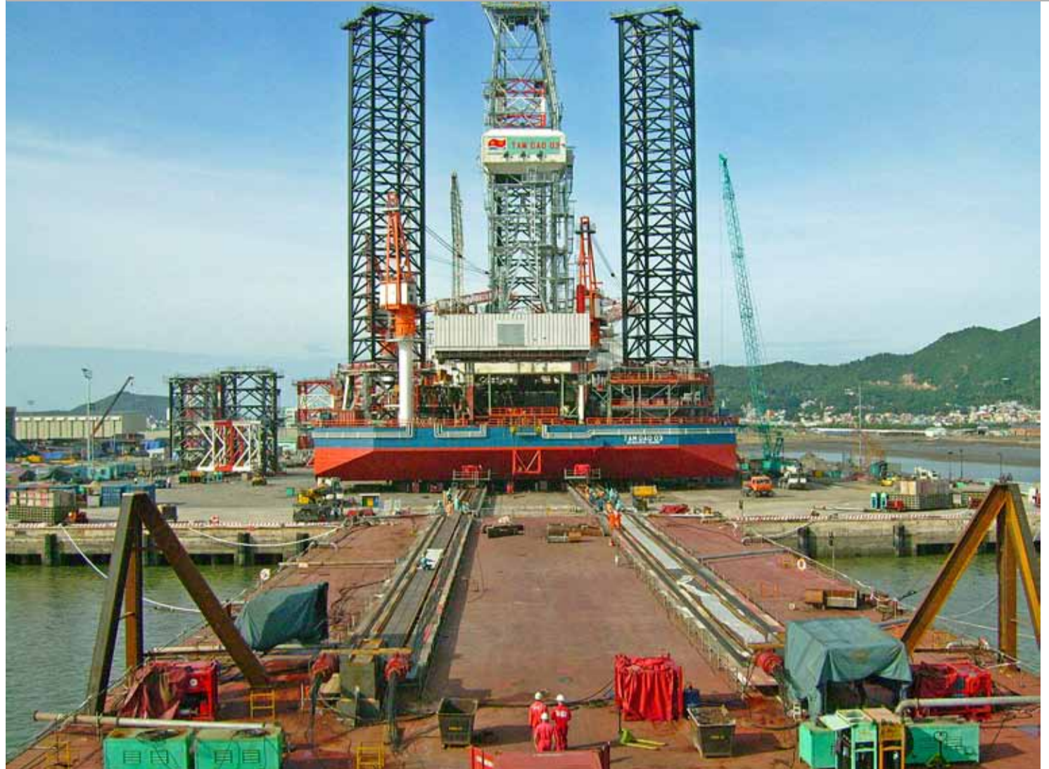
Load-out of jack-up rig 'Tan Dao 03' in Vietnam.
