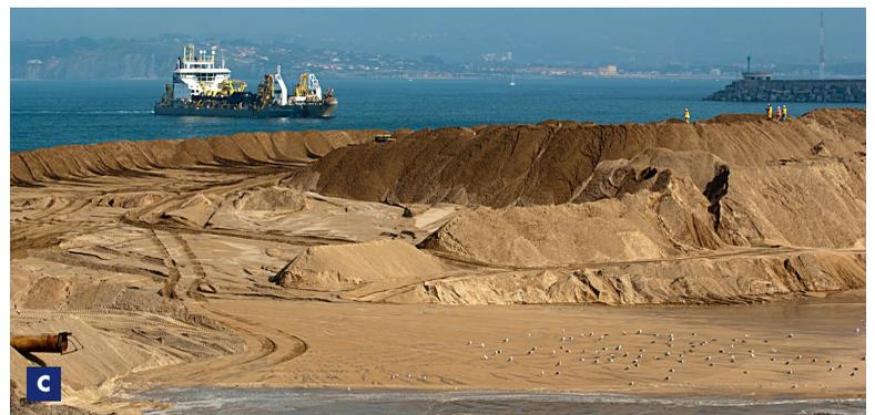
Because the dredged sand was coarser than expected (D50 200µm), a lot of wear parts had to be replaced regularly. That didn't affect the efficiency of the operations. The work for 2009, which was planned to take six months, was completed in 5 months to the satisfaction of the client, who works to tight deadlines.
