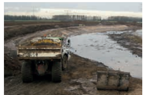
Stepped slope at Bevert Creek, Noordwaard polder
